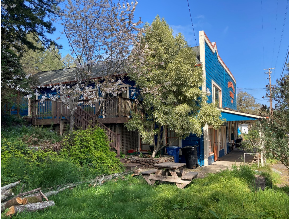
Photo 7 Southeast elevation, camera facing west
