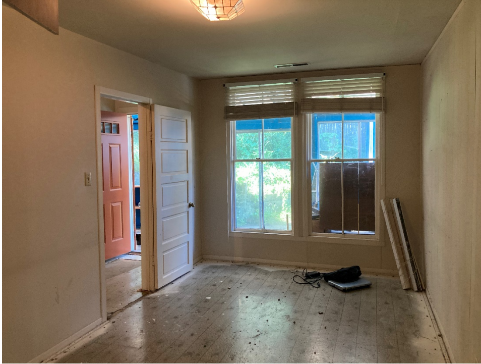
Photo 23 Interior of second floor apartment unit, bedroom, camera facing southwest
