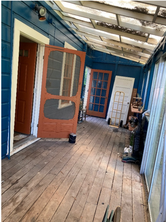
Photo 15 Rear porch of second floor apartment unit, camera facing northeast
