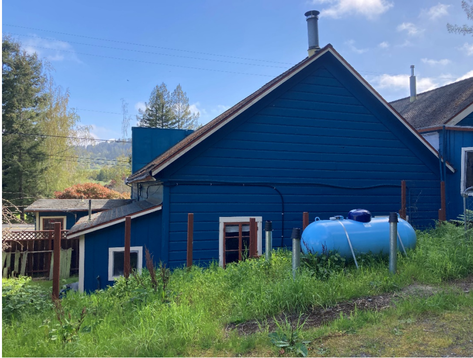
Photo 5 Rear elevation of right side, camera facing northeast
