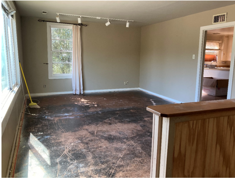
Photo 19 Interior of second floor apartment unit, living area, camera facing west
